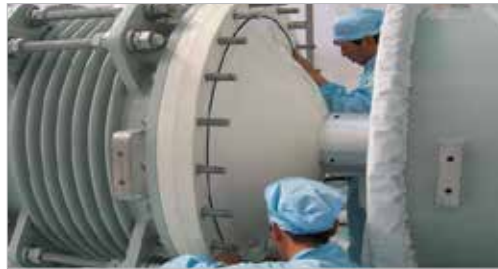
Bus Connection Work in the Wrap of Plastic Vinyl Sheet
