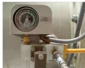
SF 6 Gas Density Transducer
