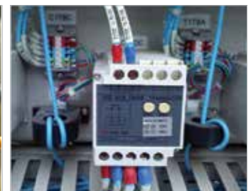
CB Operating Current Transformer
