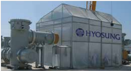
Temporary Clean Room adapted for Outdoor Type Installation
